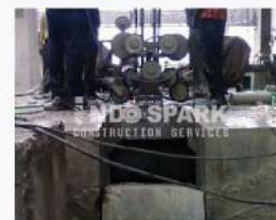
RCC Foundation after Cutting
