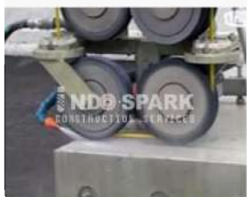
RCC Column Cutting Work
