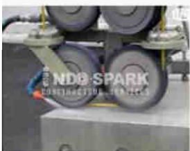
RCC Column Cutting Work
